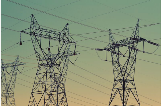
Electricity network expansion
